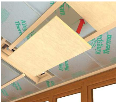
Install insulation between battens
